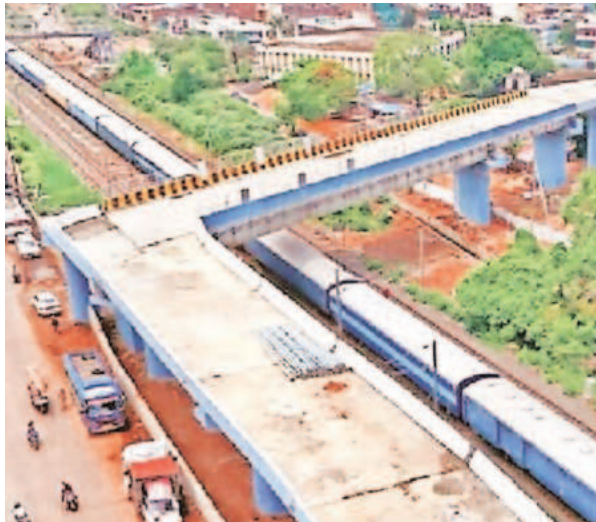
The infamous right-angle railway overbridge in Bhopal. File
