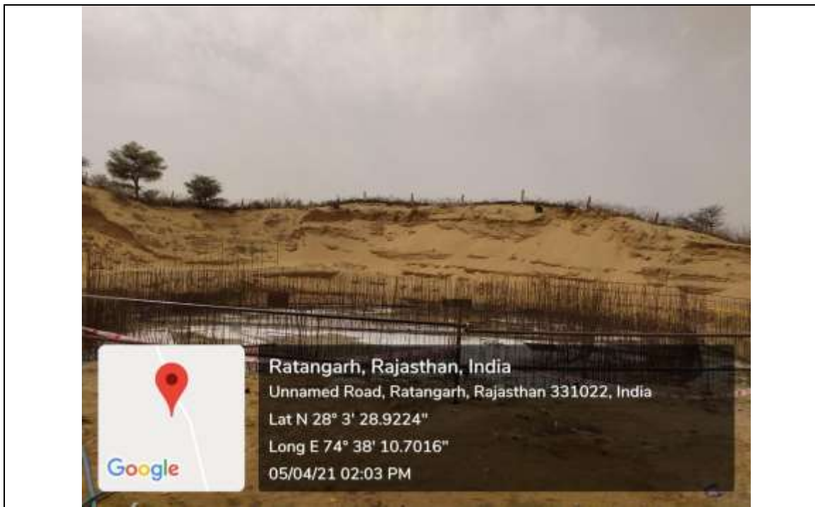
Figure 10.3A: STP-1 under construction in Ratangarh (Capacity of plant is 3.8 MLD)
