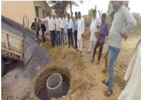
Figure 15.4(A): Magic pit construction for grey water
