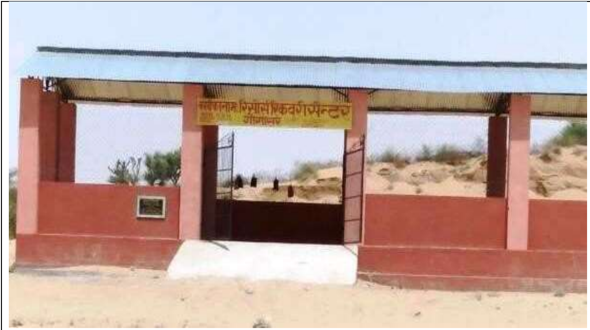
Figure 15.5(C): Garbage collection center at Gram Panchayat Gogasar after construction
