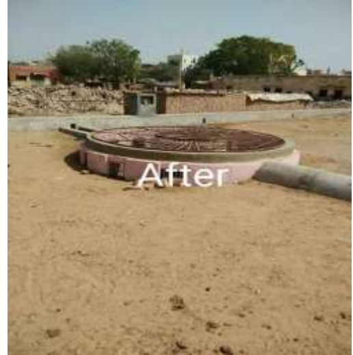
Figure 15.4(D): Status of locality after completion of work with proper drainage facilities
