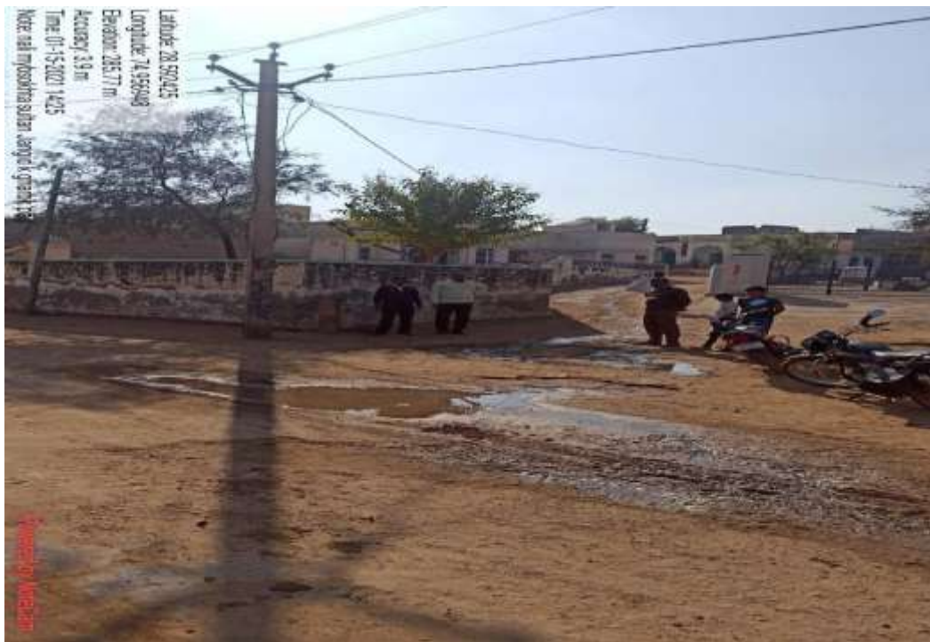
Figure 15.9D: Current status of stagnation of wastewater (Construction of drain and Community Leach pit by Connecting Multiple Household with Chamber is required)
