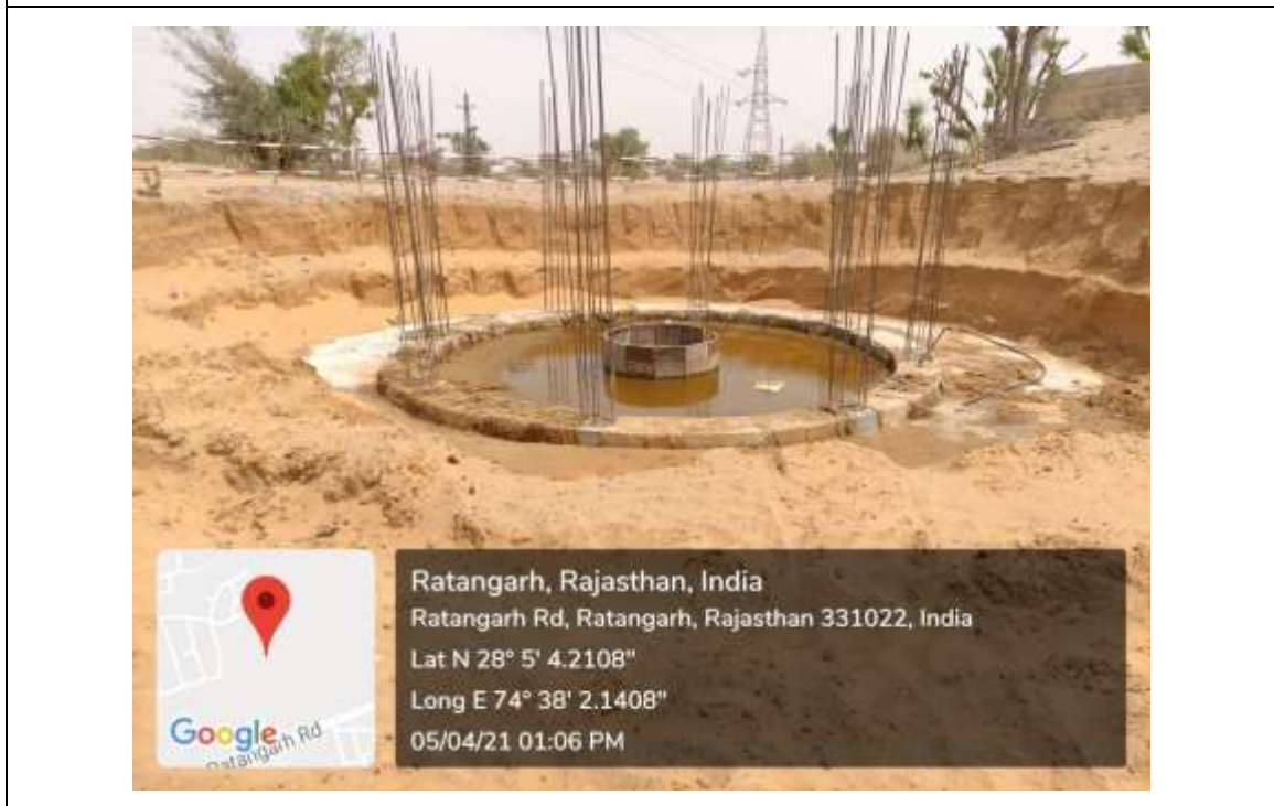
Figure 10.3B: STP-2 under construction in Ratangarh (Capacity of plant is 6.1 MLD)
