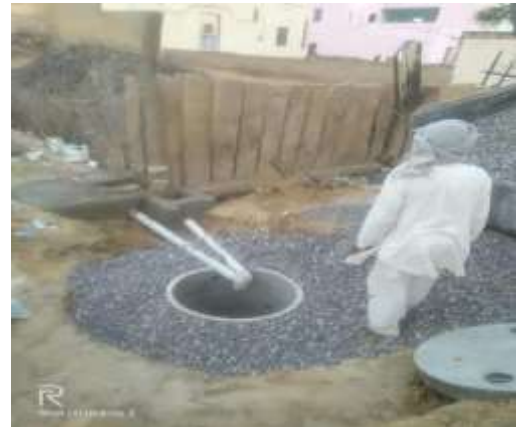
Figure 15.4(B): Construction of soak pit for grey-water management
