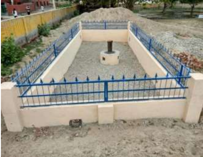
Figure 15.4(C): Recharging well for grey water management
