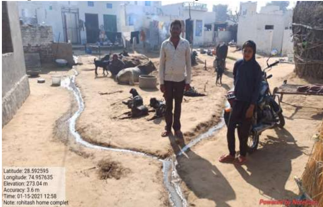
Figure 15.9C: Current status of provision of draining wastewater from individual households (Individual Soak pit is required)
