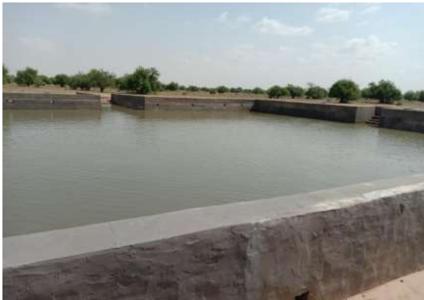
Figure 14.11: Pond Constructed under Mnerga Range Rajgarh Churu
