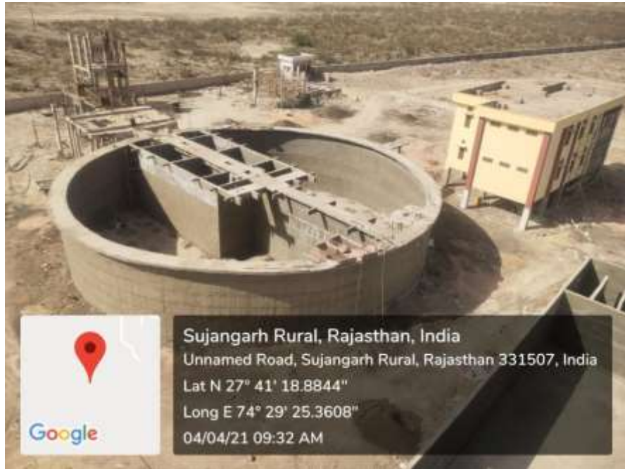
Figure 10.4A: STP-1 under construction in Sujangarh Rural (Capacity of plant is 5.5 MLD)
