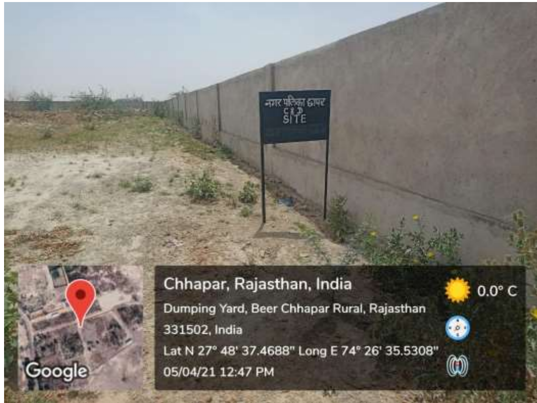
Fig. 5.2B: C&D Dumping Yard Site in Chhapar Nagarpalika, Churu
